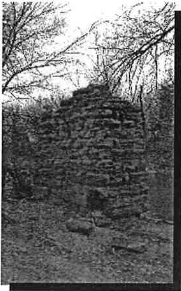
Figure 53. The old limestone trestle support on the COMED property.
