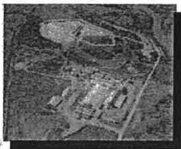
Figure 14. Aerial view of Smith-Douglass facility circa. 1965.
