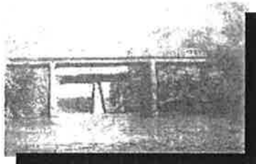
Figure 15. Former Route 23 Bridge with Santa Fe rail bridge beyond.
