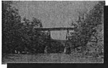
Figure 22. The dramatic, industrial bridge still in use across the Vermilion River.
