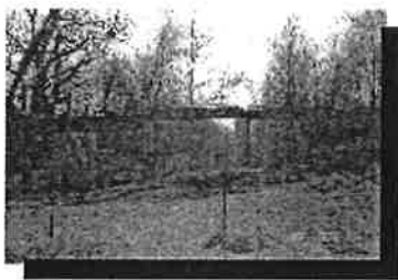
Figure 43. Abandoned rail bridge in Spring Lake Park.
