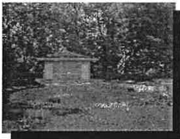
Figure 46. This public restroom's building material fits its rustic setting. It also employs a living "green roof" and a "green" septic system using plant materials.
