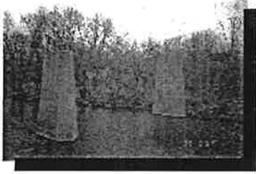
Figure 41. Existing concrete bridge supports between COMED site and St. Mary's Cemetery.
