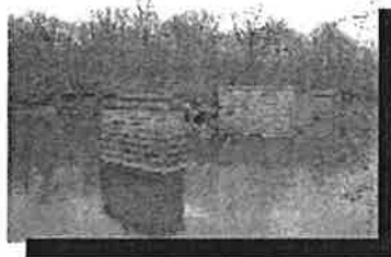
Figure 32. Those same supports could carry a pedestrian bridge today.
